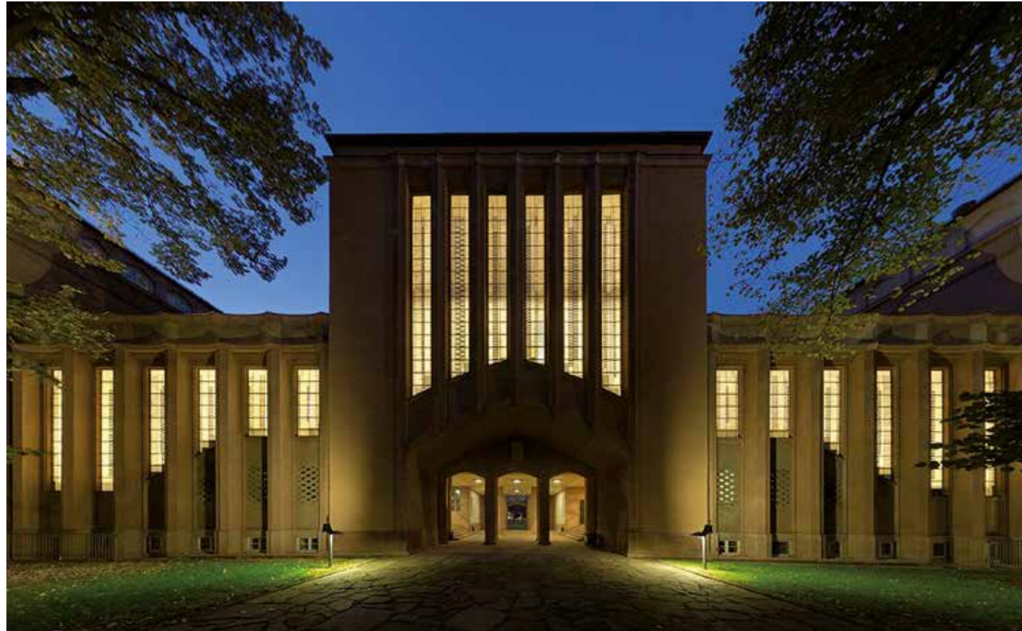
Exterior view after reconstruction
