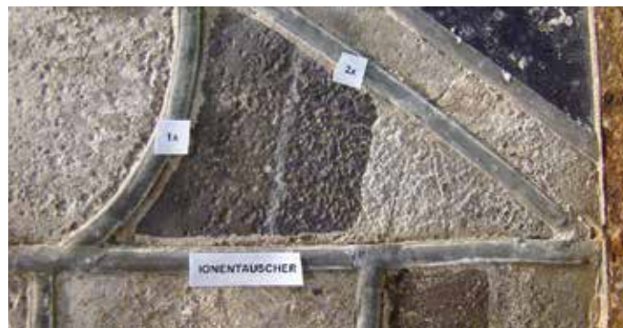
Cleaning with ion exchanger
