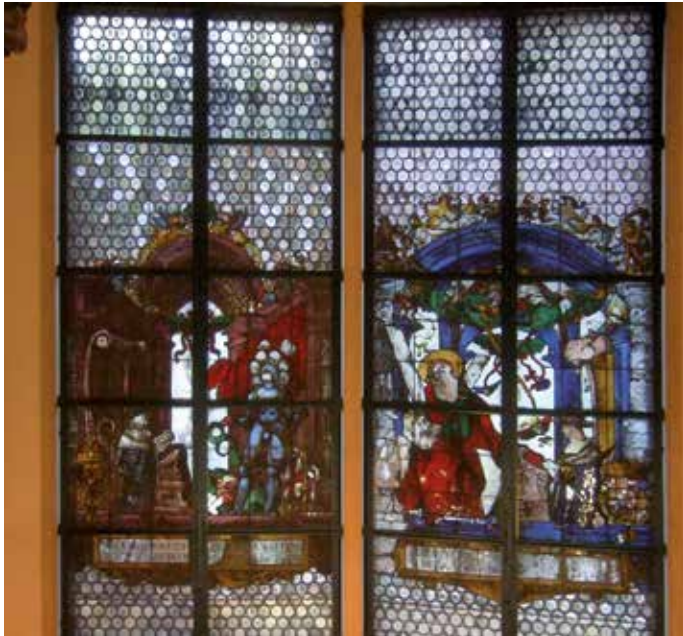
Original panes and additions after reinstallation
