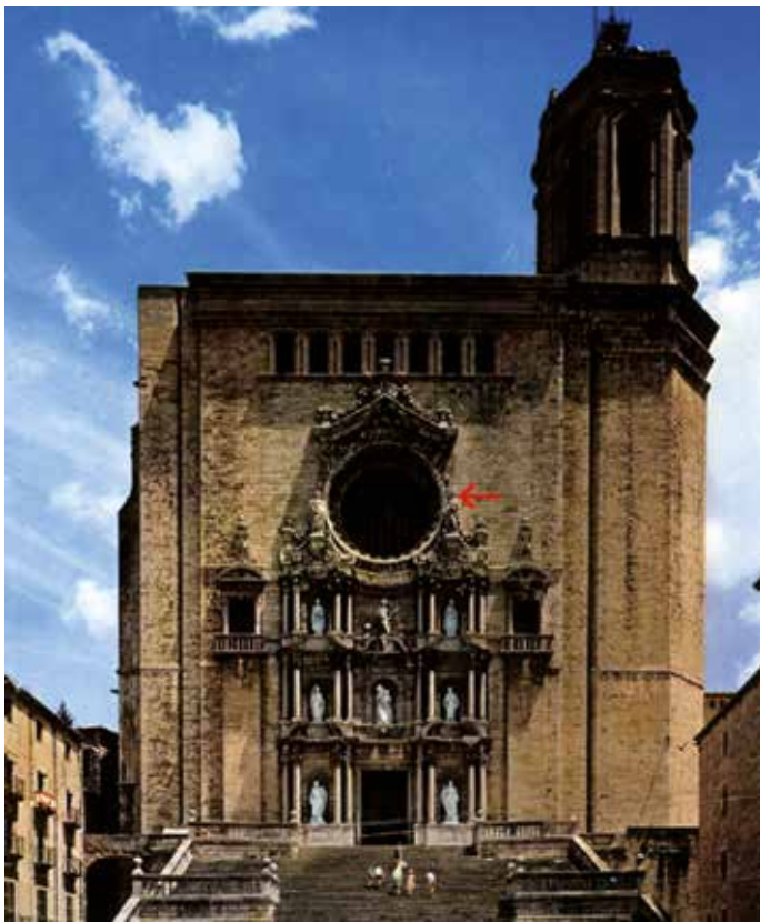
West portal with rosette, diameter approx. 8 m
